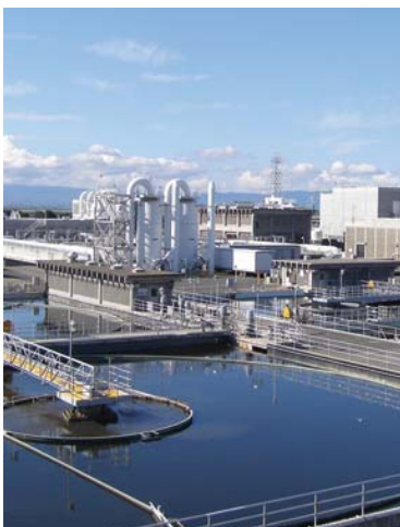
Union Sanitary District Alvarado Plant in Union City, CA
